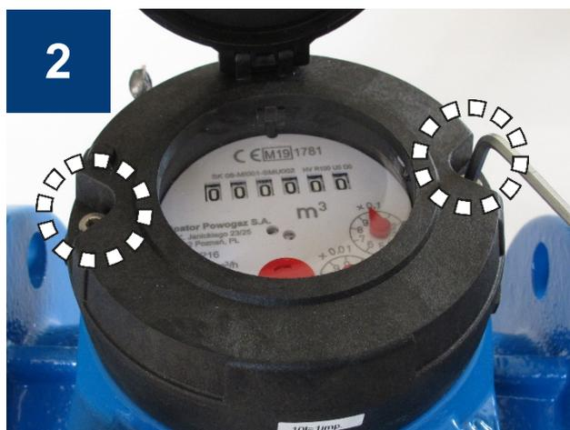
Remove the two Allen bolts and remove the counter guard assy.
